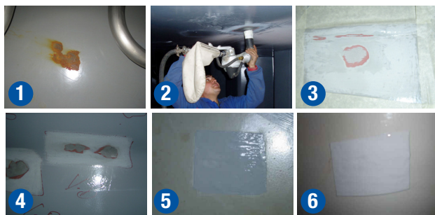
1) Rust spot 2) Vacuum blasting 3) 4) Prepped repair areas shown 5) 6) Finished MarineMend repairs
