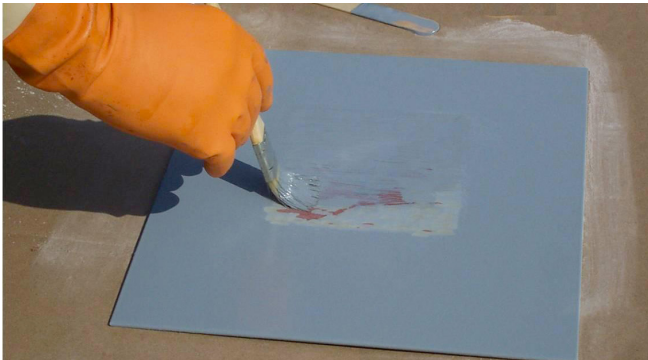
MarineMend Base Coat applied with brush.
