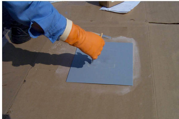
MarineMend Top Coat applied with a brush.
