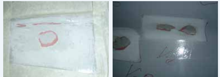
Prepped repair areas shown
