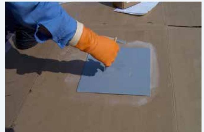
MarineMend Top Coat applied with a brush.
