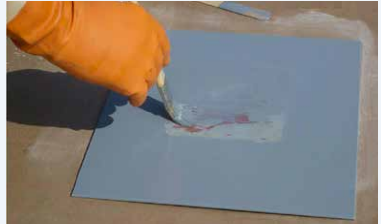
MarineMend Base Coat applied with brush.
