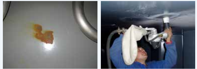
(L) rust spot (R) vacuum blasting
