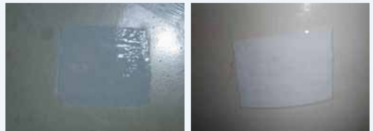
Finished MarineMend repairs
