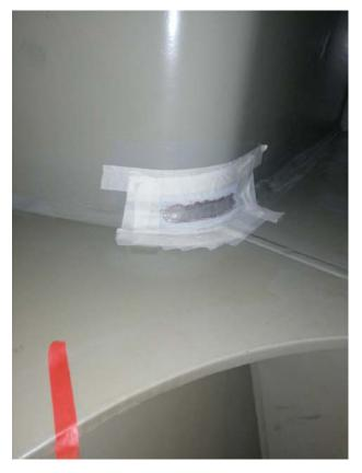
**2)** Spot grinding for small rust spots, such as pinpoint rust. Also feathering and cleaning before touch-up. Please be noted any contamination such as oil/grease should be cleaned up before the surface preparation.
