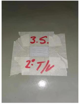
Touch-up with MarineMend repair kit (first coat Grey color). After the first touch-up is hard dry, which may be up to 24 hours depending on the temperature and air flow, sand smoothly by sandpaper before second touch-up.
